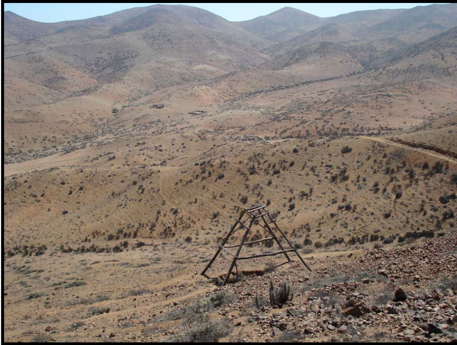
Figure 9 - Argentina Shaft and Headframe in the northern Perth Project area (photo provided by Red Metal).
